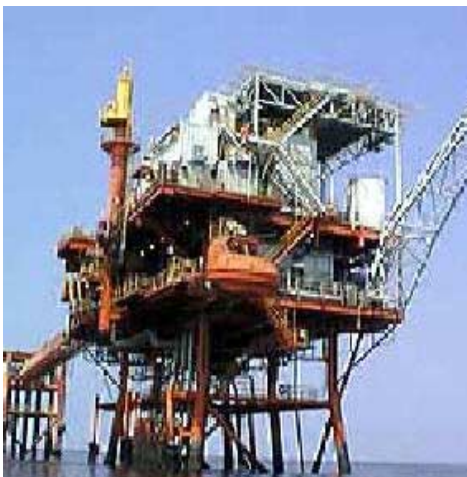
Figure 5: Inserting the wrong sand screens in oil wells once caused US$300 million of damage
